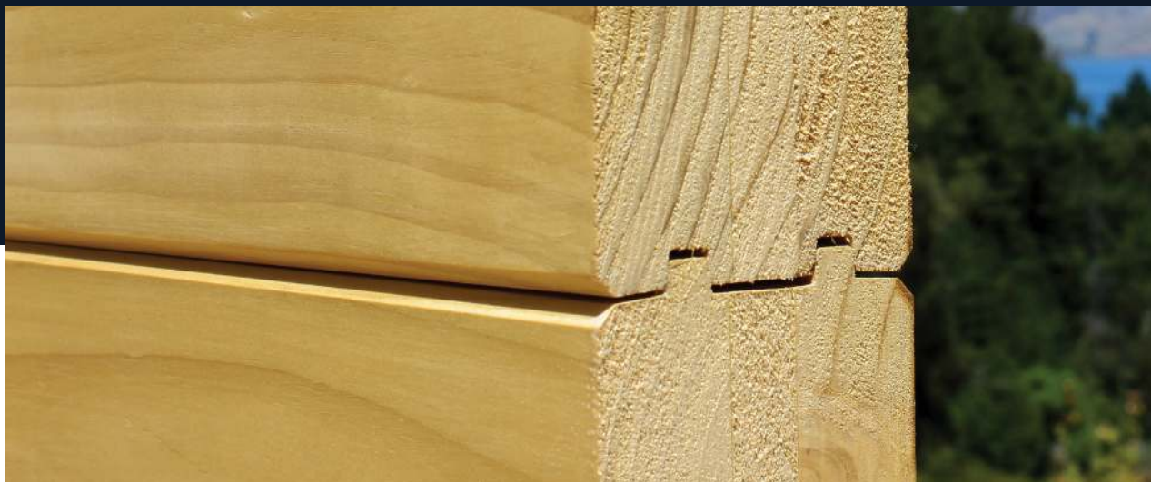
Interlocking walls (internal walls shown) in a Fraemohs Solid Timber home. Our timber provides the internal finish, external finish, insulation, and structural strength. Just wood. No trickery.
